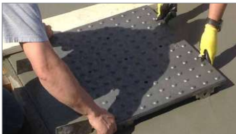
Place and press plate into fresh setting concrete.
